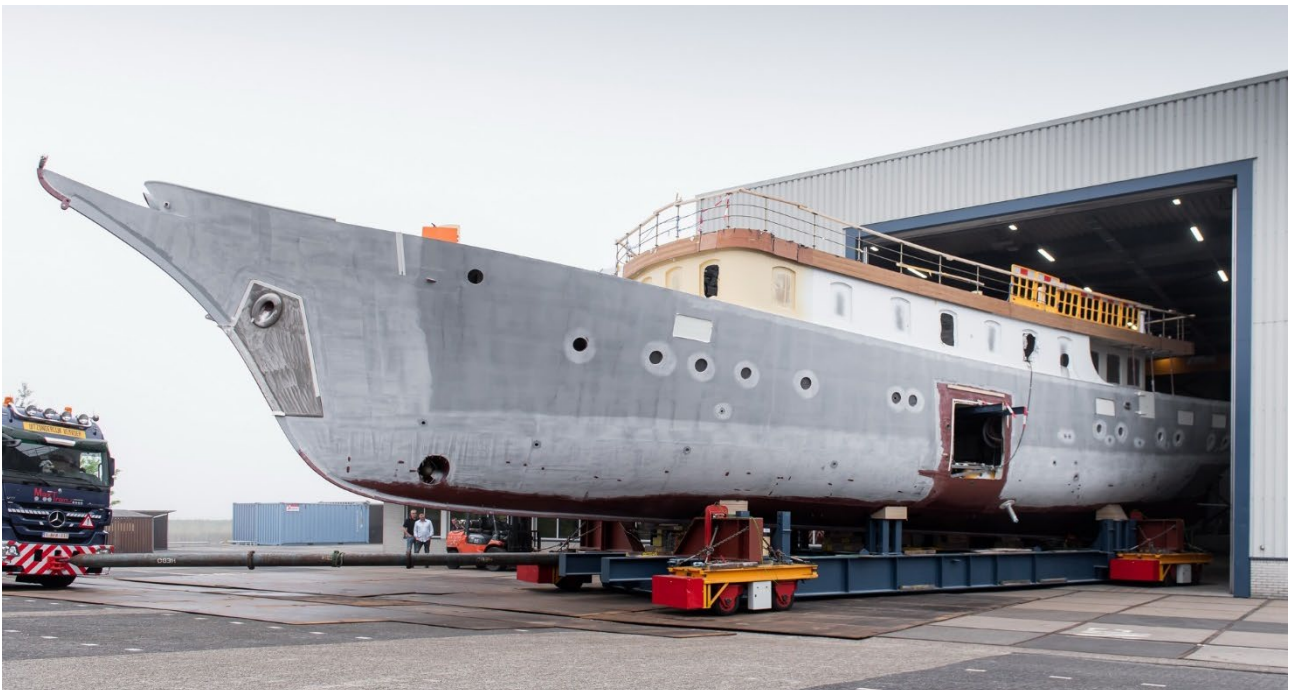
ATLANTIDE REBUILD IN PROGRESS
